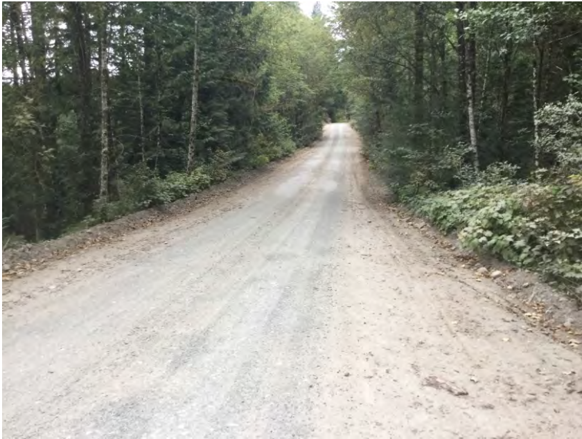
Culvert Right Approach
