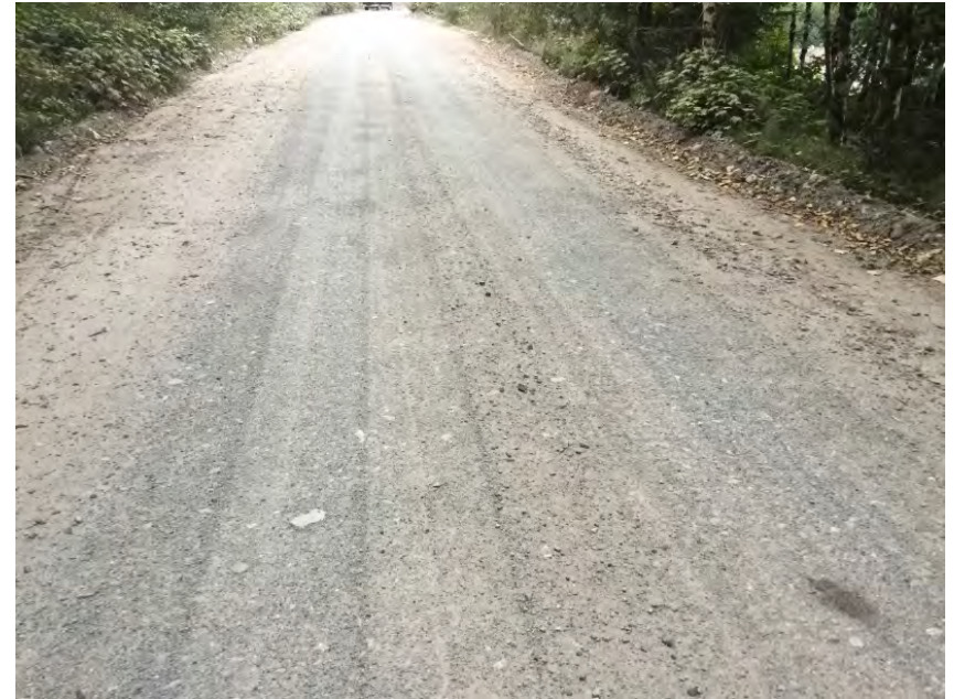
Roadway Over Culvert
