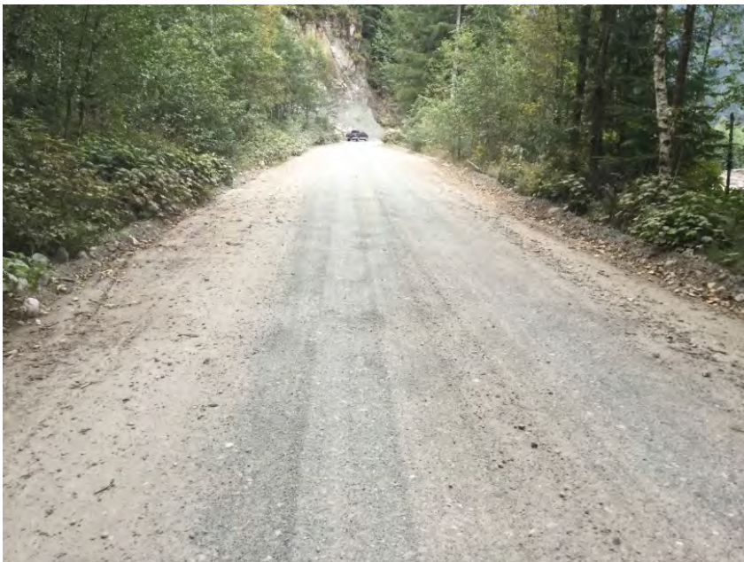
Culvert Left Approach
